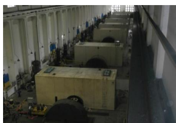
b) Internal View
