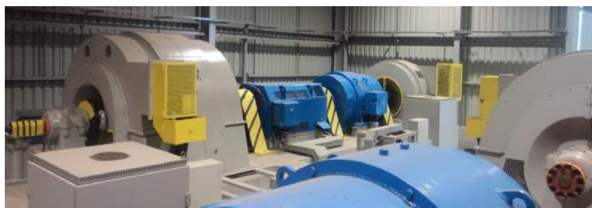
Kramer Cascade: a complex control system for a Generating Group in the testing chamber for large transformers, for the company COEMSA, in Canoas, State of Rio Grande do Sul.
